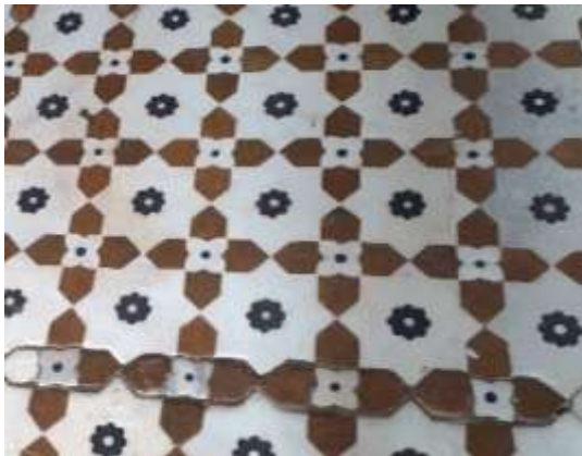
Figure 20. Inlaid floor in the interior of Jahangir's Tomb, Lahore. (Source: Captured by the author).
