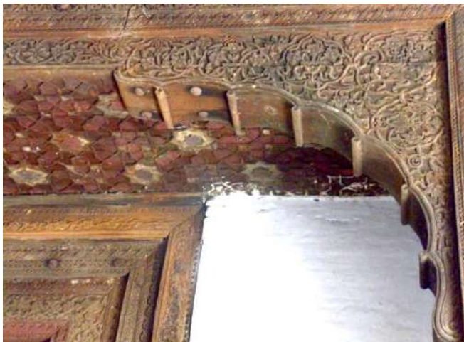
Fig. 3. Massive wooden beams supporting the roof systems.
