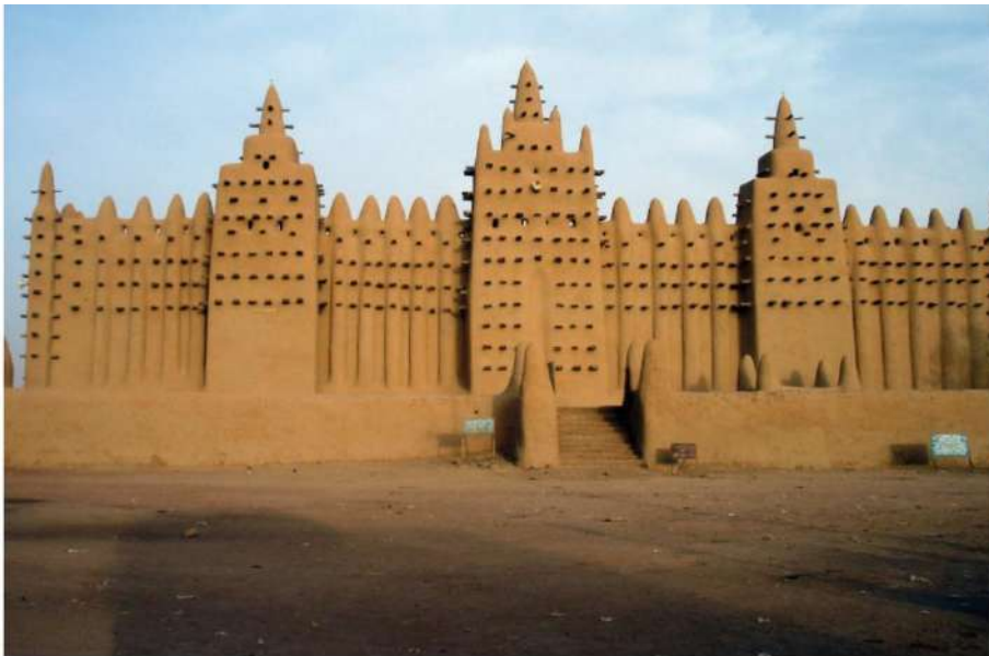
Figure 3. Façade of the Great Mosque. Source: Djenné Mosque (zamaniproject.org).
