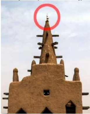
Fig. 4: Ostrich egg circled in red at the top of pillar (Source: Great Mosque of Djenné (article) | Khan Academy )
