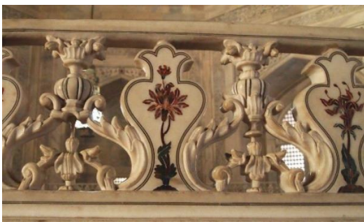
Figure 33. Balustrade Carved and Inlaid with Stones, interior of the Taj Mahal, Agra, 1648. Source: "The Mausoleum of the Taj Mahal," accessed July 24, 2019, https://www.wonders-of-the-world.net/Taj-Mahal/Mausoleum-of-the-Taj-Mahal.php .
