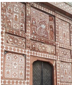
Figure 28. Still Life Motifs, White Marble Inlaid in Red Sand Stone, Exterior of Jahangir's Tomb, Lahore, 1637. Source: Picture by Sidra Liaqat.
